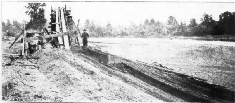
The Inhaul Path to the Plant
